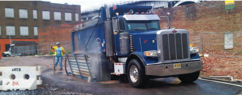
Top: Manhattanville campus construction site aerial view looking northeast with steel erection of Jerome L. Greene Science Center (center) and slurry wall panel installation around the perimeter of the site. Bottom: An innovative wheel washing system cleans truck tires and undercarriages with high volumes of recycled water, removing sediment before vehicles leave the construction site to minimize dust in the air.
